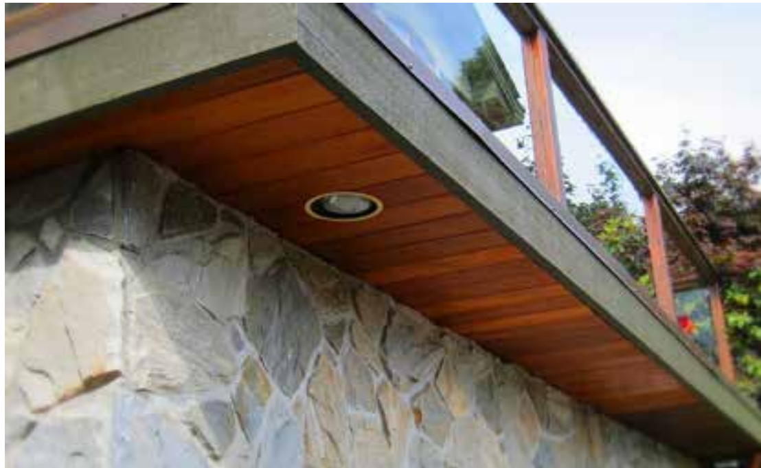
Wood Soffit System
