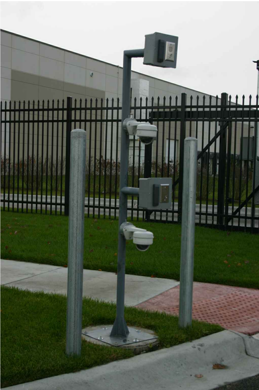
DOUBLE-GOOSENECK GATE ACCESS DETAILS
