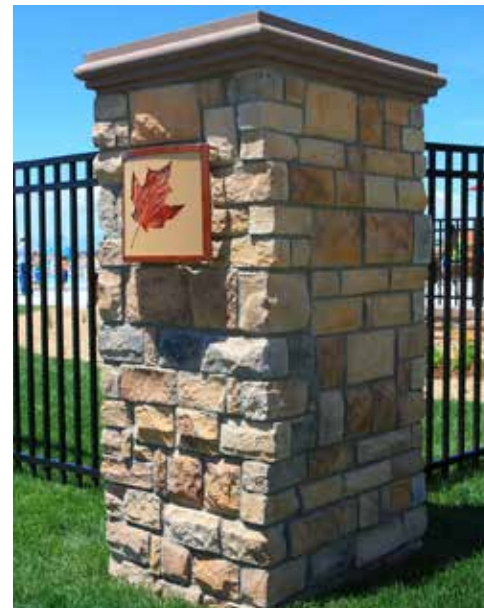
LARGE COLUMN (MIN. HEIGHT = FENCE HEIGHT + 1')
