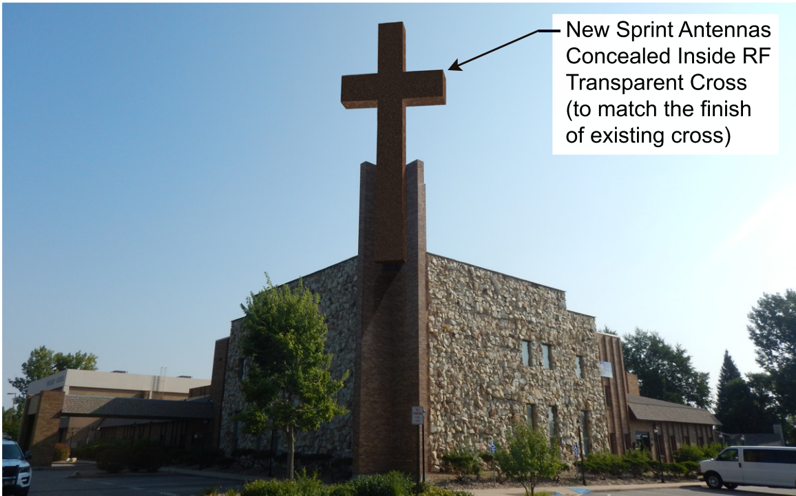
New Sprint Monopole w/ Antennas & Equipment Enclosure
