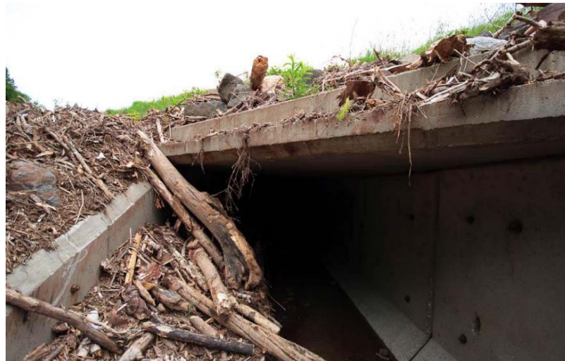
Figure 3: Debris accumulation at entrance to undersized culvert (Minnesota Department of Natural Resources, 2014).
