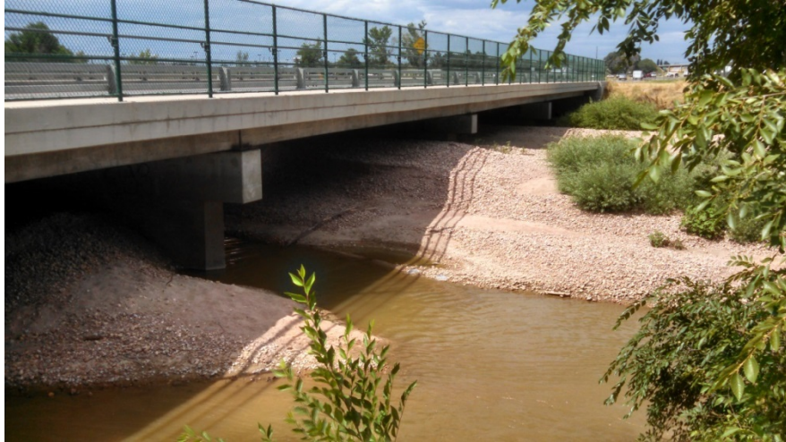
Figure 4: Sediment deposition at river crossing on Poudre River in Greeley, Colorado.
