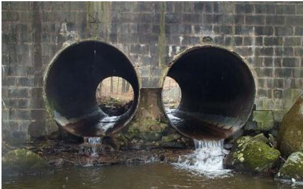
Figure 5: Perched Culverts (Connecticut Department of Environmental Protection, 2008).
