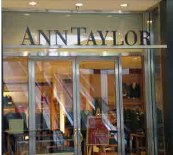
Pin-mounted letterforms are freestanding above a metal canopy,
