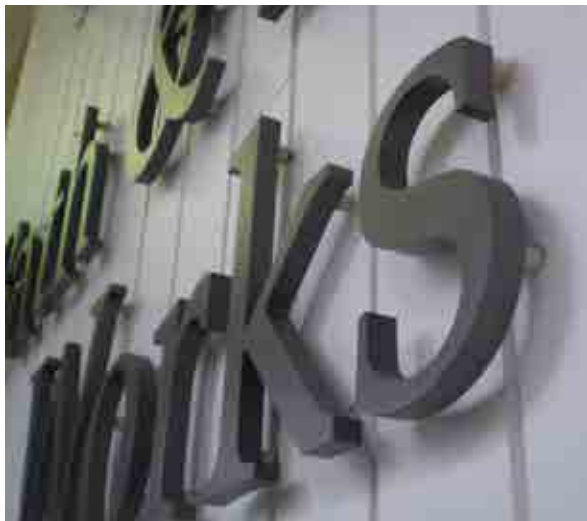
Pin-mounted letterforms are mounted off the face of wall
