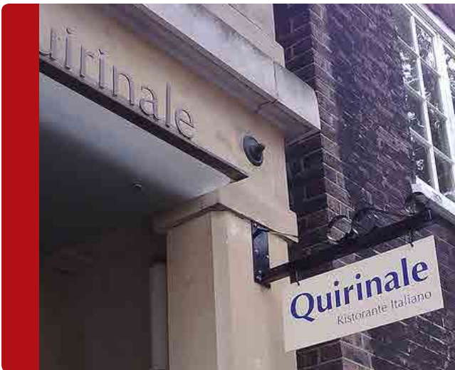
Bracket attaching awning frame system to brick should also be the same color as frame and storefront
