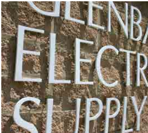
Metal letterforms are pin-mounted off brick storefront
